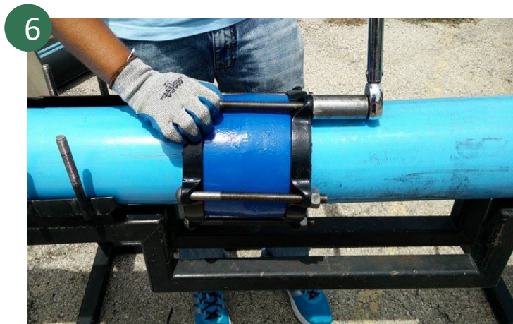
Pressurize the line, check the leakage, and re-torque if necessary.
