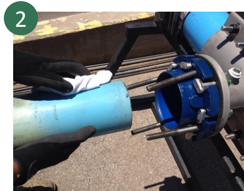
2 Thoroughly clean the pipe end where the adapter will be installed.
