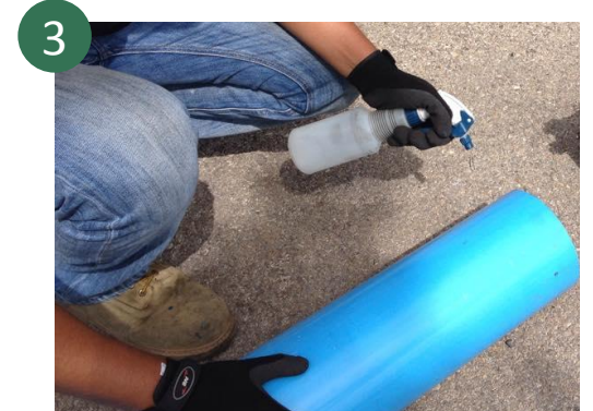
3 Lubricate pipe end and coupling gasket with a soapy solution.
