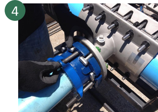
4 Hand tighten gland bolts and stab plain-end pipe into coupling.
