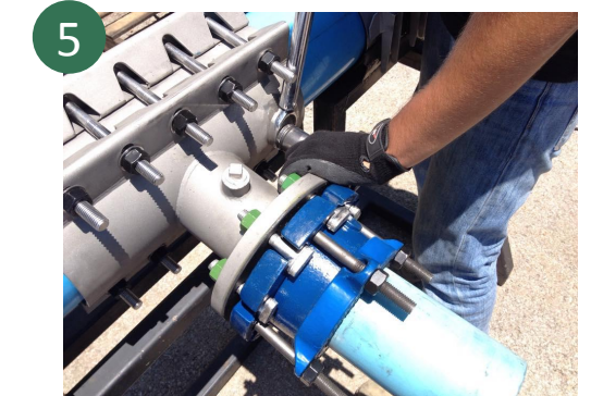
5 Evenly tighten flange bolts in a radial pattern and proceed to evenly tighten gland bolts to the recommended torques.
