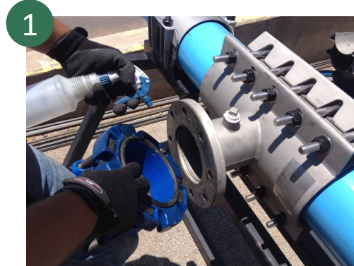
1 Lubricate flange o-ring and gasket and connect adapter flange to flanged pipe or fitting using T-bolts.
