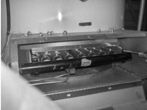
Step 7: Remove manifold bracket screws
