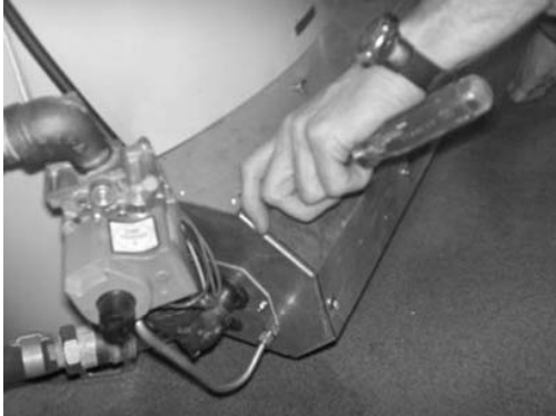
Step 1: Remove burner box cover screws
