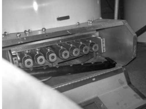
Step 8: Remove manifold from Burners
