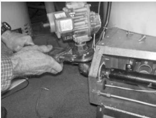
Step 5: Disconnect and Remove Gas Valve
