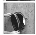
NOTE: To insure minimum water migration, center the water stop in wall by cutting equal lengths from each end of the sleeve, except as noted below.
