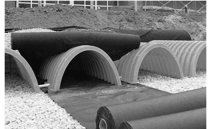
Place two continuous layers of ADS Woven fabric between the foundation stone and the isolator row chambers, making sure the fabric lays flat and extends the entire width of the chamber feet. Drape a strip of ADS non-woven geotextile over the row of chambers (not required over DC-780). This is the same type of non-woven geotextile used as a separation layer around the angular stone of the StormTech system.
