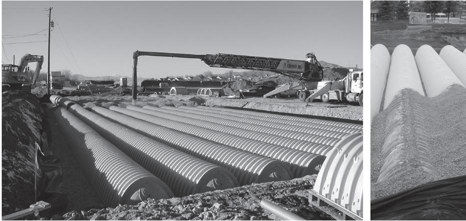
Initial embedment shall be spotted along the centerline of the chamber evenly anchoring the lower portion of the chamber. This is best accomplished with a stone conveyor or excavator reaching along the row.
