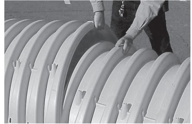
Continue installing chambers by overlapping chamber end corrugations. Chamber joints are labeled “Lower Joint – Overlap Here” and “Build this direction – Upper Joint” Be sure that the chamber placement does not exceed the reach of the construction equipment used to place the stone. Maintain minimum 6” (150 mm) spacing between rows
