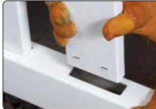
Quickly lock rails and pickets in place.
