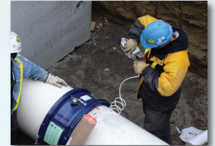
The Hymax 2000 offers an efficient range adjustable pressure assisted hydraulic sealing system. The gasket is compounded of an NSF 61 registered EPDM material.
