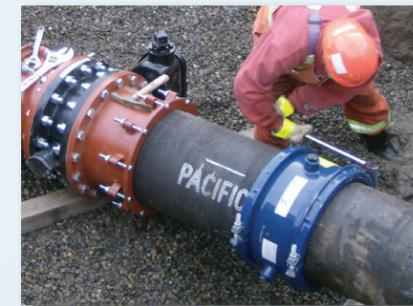
The large diameter Hymax 2000 is a stab type coupling requiring no disassembly. Installer simply adjusts gasket and tightens two bolts on each end of the coupling to required torque. All work is performed from topside of the coupling, eliminating need for extra excavation and under-dig for the wrench.
