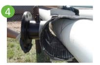
Position flanged (or MJ-Mechanical Joint) half of sleeve on pipe making sure outlet is properly aligned with branch-line to be connected. Make certain that the tapered ends of the complete circle gasket are smooth against the pipe. Never position so that rotation of sleeve is required.
