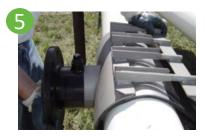
Position back half of sleeve over the tapered ends of the gasket being careful not to fold or roll the edges under themselves. Locate Bolts between fingers on the flanged half of sleeve.
