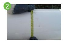
Check the main outside diameter (OD) and confirm that it falls within the tapping sleeve pipe OD range.
