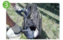
Lubricate pipe and gasket with soap/water solution. **Do not use grease or pipe lubricant.**
