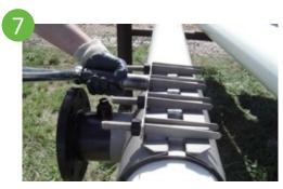
Begin tightening bolts in sequence, beginning at the center of the sleeve and alternating on both sides. The gap between the two halves must be of equal distance when sleeve is fully tightened.
