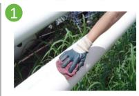
Thoroughly clean the pipe so surface is smooth and free of dirt and other debris.
