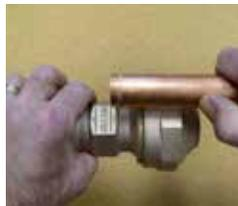
**2. INSERTION LENGTH:** Put the fitting beside the pipe and note the length of the pipe to be inserted (use your thumb or marker as a guide.)
