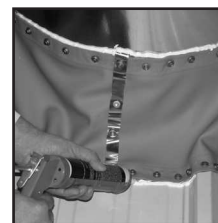
6. Apply sealant to all seams.
