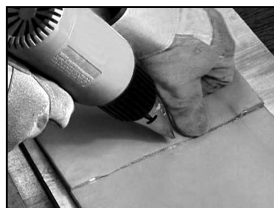
3. Apply heat and press firmly to seal edges.
