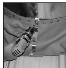
5. Fasten through top of termination strip, Dekstrip, and back of strip with Scots® fasteners or rivets.
