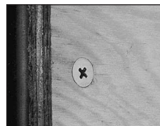
Plywood to steel or wood studs.
