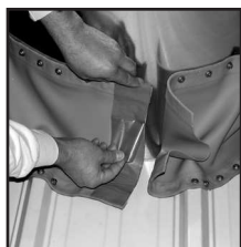
2. Remove film from top of splice tape.
