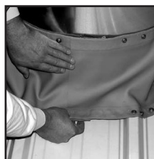
3. Overlap top piece of Dekstrip and press onto tape.
