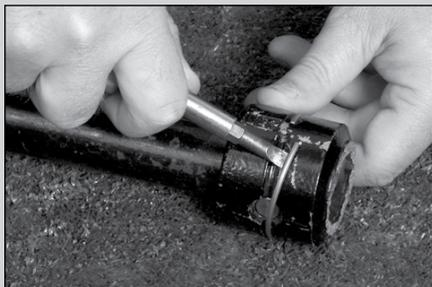
**1** The hydrant can be restored to service without removing the bonnet or valve rod assembly by using the Traffic Repair Kit, which includes items 26-31, plus item 49, shown in drawing on Page 2. First, remove broken Valve Rod Coupling halves, Pins and Retaining Rings from Upper and Lower Valve Rod ends.
