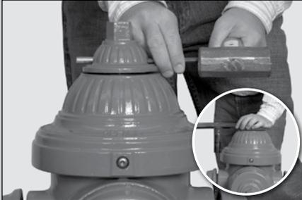
**1** Drive out Operating Nut Locking Pin from rounded side of Operating Nut. Remove Operating Nut, while taking care not to lose Operating Nut Seal, which is located inside the Operating Nut. With an 1/8" Allen wrench, loosen Hold Down Nut Screw – then remove Hold Down Nut using the Combination Spanner Wrench by turning counterclockwise.
