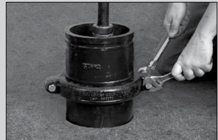
**5** Install Extension Standpipe Coupling with stainless steel Bolts & Nuts, so the grooves in both the Lower Standpipe and Extension are engaged equally, and bolts are tightened to 50 ft-lbs torque, and the space between ends of coupling are equal on both sides of hydrant.
