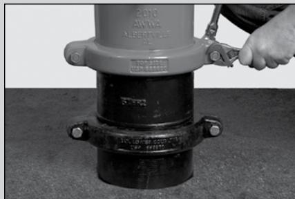
**7** Reassemble frangible Standpipe Coupling around lip of Upper Standpipe and groove in the Extension. Make certain that there is uniform engagement all around— then, carefully tighten the Coupling Bolts & Nuts to 50 ft-lbs torque, and the space on each side is equal.
