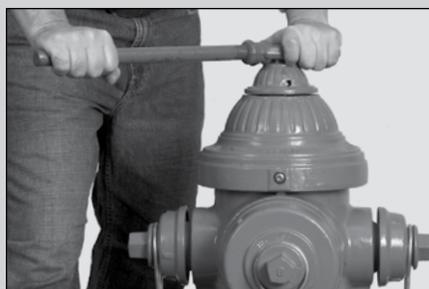
**6** Slowly turn the Operating Nut in the closing direction, lowering the hydrant top section over the bottom section. Then, position the hydrant to face the proper direction. When the top section is aligned with the bottom section, continue to close until snug.
