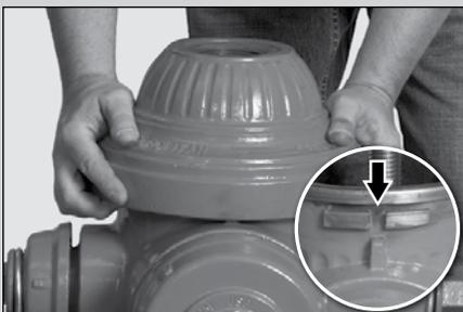
**7** Replace the Bonnet Seal. Grease threads on Upper Valve Rod. Replace the Bonnet, turning clockwise into locked position. Next, grease the threads on Bonnet Locking Screw and reinstall. Be certain that the Bonnet is centered, so locking screw sets in the "V" of the locking slot in the Upper Standpipe.
