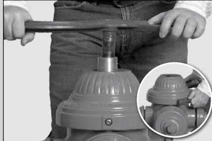
**2** Using socket of Combination Spanner Wrench or 3/4" thinwall socket, remove Travel Stop Nut. Remove Revolving Nut – turn in operating direction of hydrant. It is not necessary to separate the Anti-friction Bearing from Revolving Nut. Using a 7/32" Allen wrench, remove Bonnet Locking Screw. With the Combination Spanner Wrench, rotate Bonnet 22.5° (1/16 turn) counter-clockwise. As lugs disengage, lift the Bonnet off the Valve Rod.
