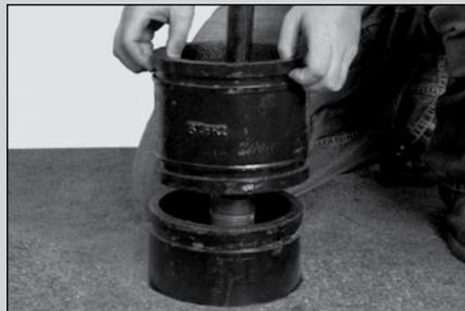
**4** Clean grooves in Lower Standpipe and Extension section. Install the Extension Coupling Gasket in groove on the bottom of the Extension. Either grease or gasket cement may be applied to keep it in place. Position the Extension over the Lower Standpipe.
