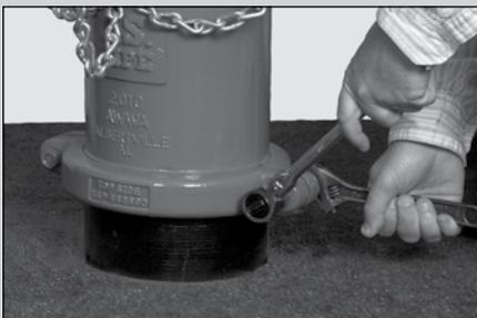
**4** Retighten the Bolts and Nuts on the frangible Standpipe Coupling. Make sure to carefully tighten them to 50 ft-lbs torque, and the spaces between the ends of each coupling half are equal.
