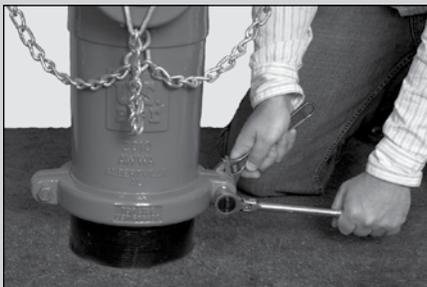
**2** Loosen, but do not completely disassemble the frangible Standpipe Coupling Bolts & Nuts.
