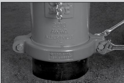
**8** Carefully tighten the Coupling Bolts & Nuts to 50 ft-lbs torque, and the space on each side is equal. Operate hydrant and check for leaks.
