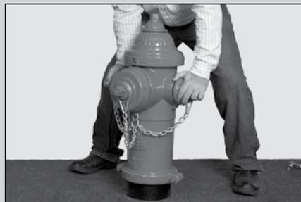
**3** Rotate the hydrant to the desired position.
