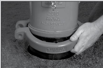
**7** Assemble frangible Standpipe Coupling, making certain the bottom of the coupling is in its groove and that the top half of the coupling is uniformly engaged on the shoulder of the Upper Standpipe.
