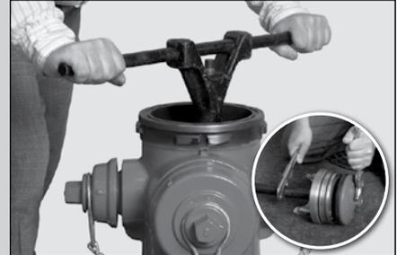
**3** Remove Bonnet Seal. Using Seat Removal Wrench, unscrew the Valve Rod and Main Valve assembly, including bronze Seat Ring, by turning counterclockwise, and removing it as a unit. Holding Lower Valve Rod with a wrench, remove the Valve Bottom Plate.
