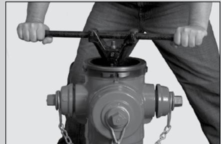
**6** Reversing the above procedure, reinstall the Valve Rod and Main Valve assembly, fully threading it into the Seat Ring. To check for any leaks after being reinstalled, pull up on the Valve Rod to close the Main Valve – then, slowly open the auxiliary hydrant control valve to pressurize the elbow. Make sure seal is tight.
