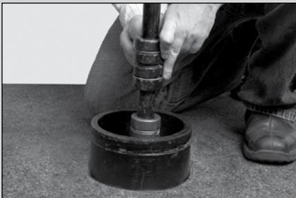
**3** Install Rod Extension between Upper and Lower Valve Rods, making sure that the non-frangible Extension Rod Coupling (without break groove) is below, and the frangible Valve Rod Coupling (with groove) is above. Be sure to reinstall Dampener ring between Extension and Frangible Couplings. Replace all Pins and secure each with stainless steel Coupling Retainer Rings.
