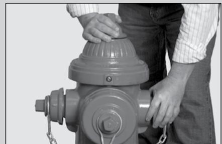
**9** Check pressure tightness of reassembled parts by following steps 2, 3 & 4 of AWWA certified inspection procedure. Following that, open the hydrant, allowing water to flow again. Close and check for proper drainage. If no problems are evident, the hydrant is already closed and considered back in service.
