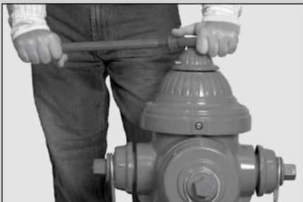
**1** Open the hydrant Main Valve three turns.
