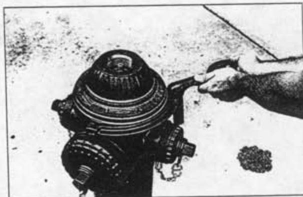
12. With combination spanner wrench, rotate bonnet 22.5 degrees (1/8 turn) counterclockwise. Bonnet lugs will disengage.
