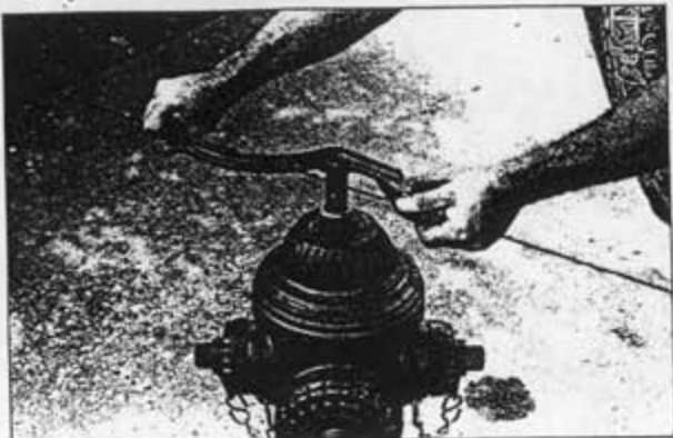
7. Using socket of combination wrench or 3/4" thinwall socket, loosen travel stop nut #5.
