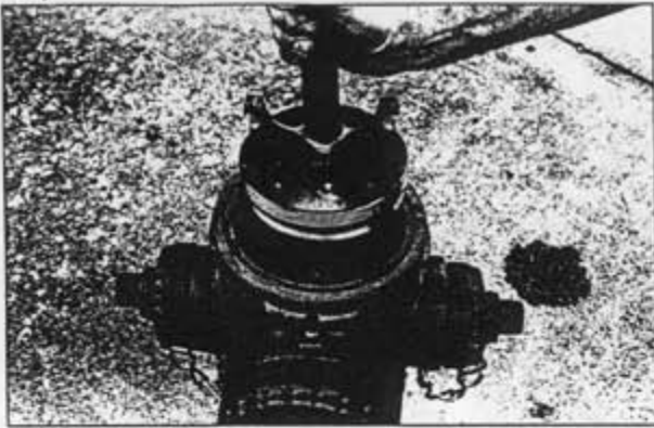
23. Reversing above procedure, reinstall valve assembly, fully threading it into the subseat. You may pull up on rod, closing valve, and opening auxiliary valves to pressurize the elbow and check for any leaks.
