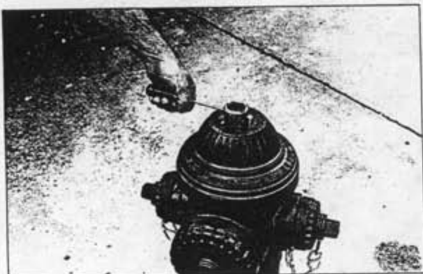
9. Loosen revolving nut #13 turning in opening direction of hydrant (it is not necessary to separate anti-friction bearing #47 from revolving nut).
