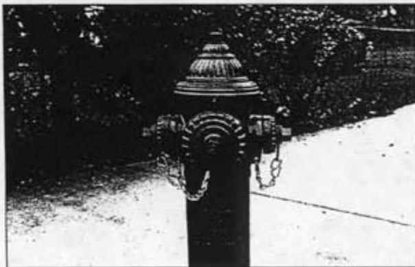
27. Hydrant closed and back in service.
