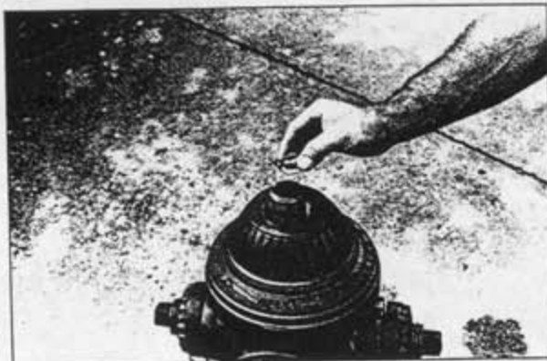
8. Remove travel stop nut #5.
