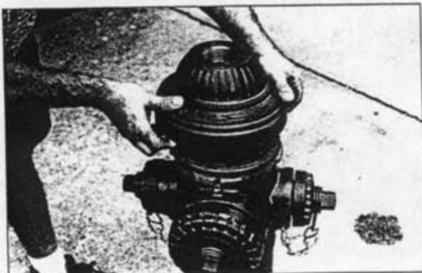
13. Lift bonnet straight up and off the operating rod.
