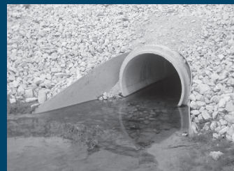
Contech End Sections are often used on concrete pipe. They can be used on both the bell and spigot end.
