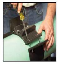
3. Position belt around pipe and secure all segments by tightening all bolts with standard screw driver or allen head (Model AZ).
