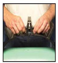
2. Pre-assemble segments by inserting bolts through spacer segments and hand tightening nuts. Leave one segment open so you can position the "belt of segments" around the pipe.
