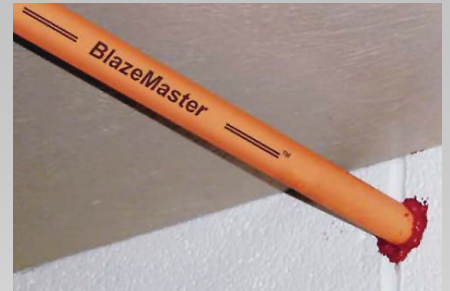
2-Hour Fire-Rated Through Penetration Firestop for Single Plastic Pipe through Concrete Walls using BlazeMaster Caulk & Walk
