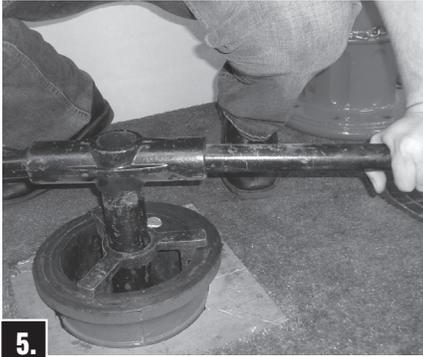
**5.** Tighten Main Valve to 100-150 ft-lbs. Turn on water at the Gate Valve and remove Wrench from Stem by removing Clevis Pin.
