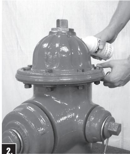
**2.** If oil is low, use a small funnel to add MUELLER Hydrant Lubricant.
