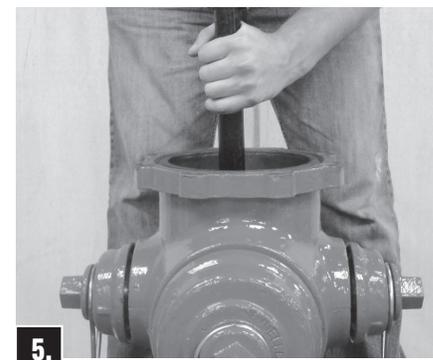
**5.** Lower Main Valve into the Barrel. Lower Support Arm and tighten Thumb Screw. Carefully thread main valve assembly clockwise into the base of the Hydrant. Hand tighten.
