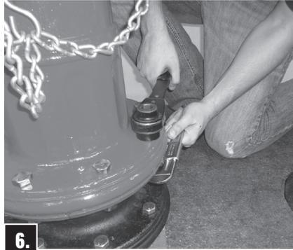
**6.** Reassemble Upper Stem to Lower Stem. Place Upper Barrel in place and reassemble Traffic Flange.\* Tighten Bolts to 60 ft-lbs.
