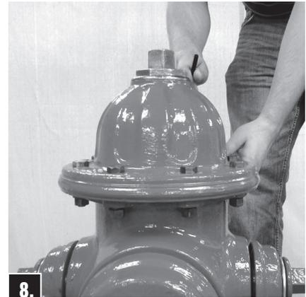
**8.** Remove Oil Filler Plug in side of Bonnet. Pour MUELLER Hydrant Lubricant into Oil Reservoir until it is level with Oil Filler Plug Hole. Replace Oil Filler Plug (see Lubrication section on page 8).
