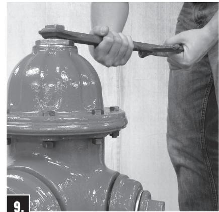
**9.** Turn Operating Nut in closing direction to make sure Main Valve is closed tightly, then turn in opening direction approximately 1/4 turn to relieve tension on operating mechanism.
