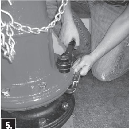
**5.** Attach Upper Barrel with new Traffic Flange Halves (with bevel on outer edge downward) and Bolts; being sure Traffic Flange O-ring\* is in groove in Upper Barrel. Tighten Bolts to 60 ft-lbs.
