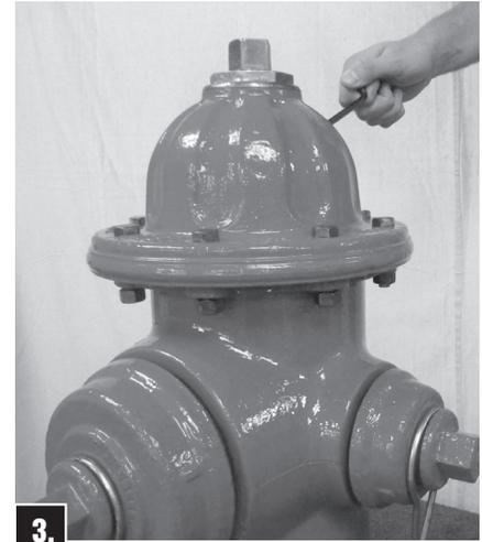
**3.** When oil is level with Oil filler Plug Hole, replace Oil Filler Plug.
