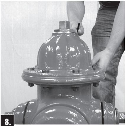
**8.** Remove Oil Filler Plug in side of Bonnet. Pour MUELLER Hydrant Lubricant into Oil Reservoir until it is level with Oil Filler Plug Hole. Replace Oil Filler Plug (see Lubrication section on page 8).
