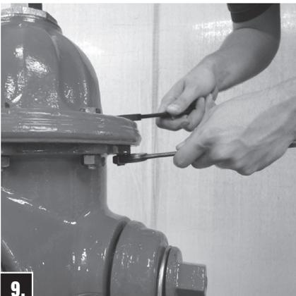
**9.** Torque Bonnet Bolts to 40-80 ft-lbs. Torque Hold-Down Nut to 200-300 ft-lbs. after Bonnet Bolts are tight. Open Gate Valve. Unscrew one Hose Nozzle Cap slightly to bleed air. Open Hydrant fully. Tighten Hose Nozzle Cap when water starts flowing and check all flange connections for leaks. Turn Operating Nut to fully closed position and remove Hose Nozzle Cap to allow Barrel to drain. Replace Hose Nozzle Cap.
