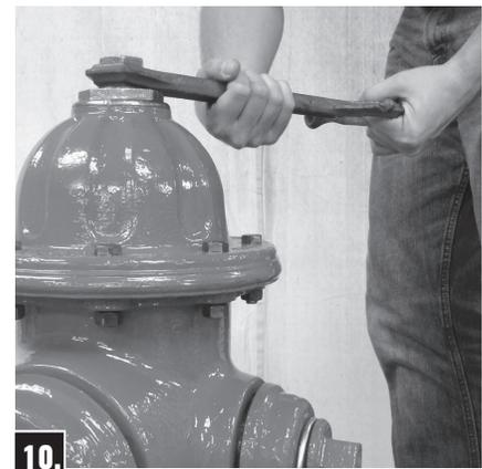
**10.** Turn Operating Nut in closing direction to make sure Main Valve is closed tightly, then turn in opening direction approximately 1/4 turn to relieve tension on operating mechanism.
