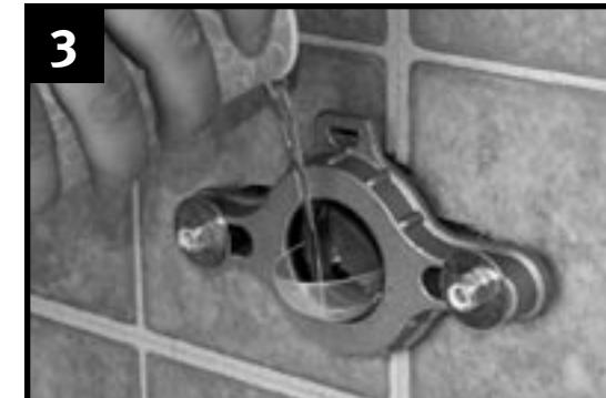
Clean face of existing wall flange then install the brass flange with the clear inspection disc. Slowly pour water into the drain.
