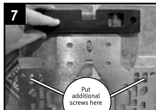
Level the bracket then mark, drill and install two additional plastic anchors and screws. If pre-existing bearing rods can be used, screws are not necessary.
