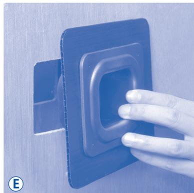
**7A.** Place interior flange over tube and screw flange in four corners, providing interior surface is other than brick or block. Caulk all edges. If interior surface is brick or block, simply caulk with Liquid Nails® as a final step.
