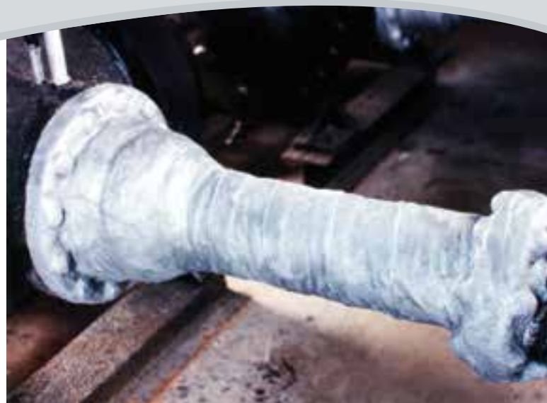
A sweating meter run pipe protected with Wax-Tape® #2A wrap demonstrates the wrap's ability to protect in wet conditions.
