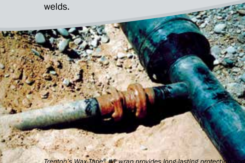
Trenton's Wax-Tape® #1 wrap provides long-lasting protection and is compatible with many types of materials, such as steel, ductile iron and PVC.
