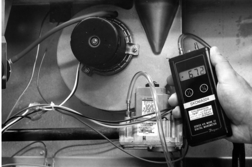
FIGURE 16 TYPICAL HOSE CONNECTION TO LINE PRESSURE TAP
