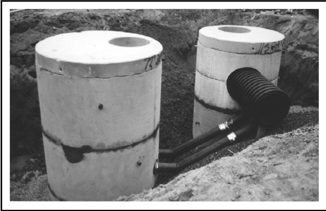
Figure 5.1: BaySeparator™ Installation at a Typical Site
