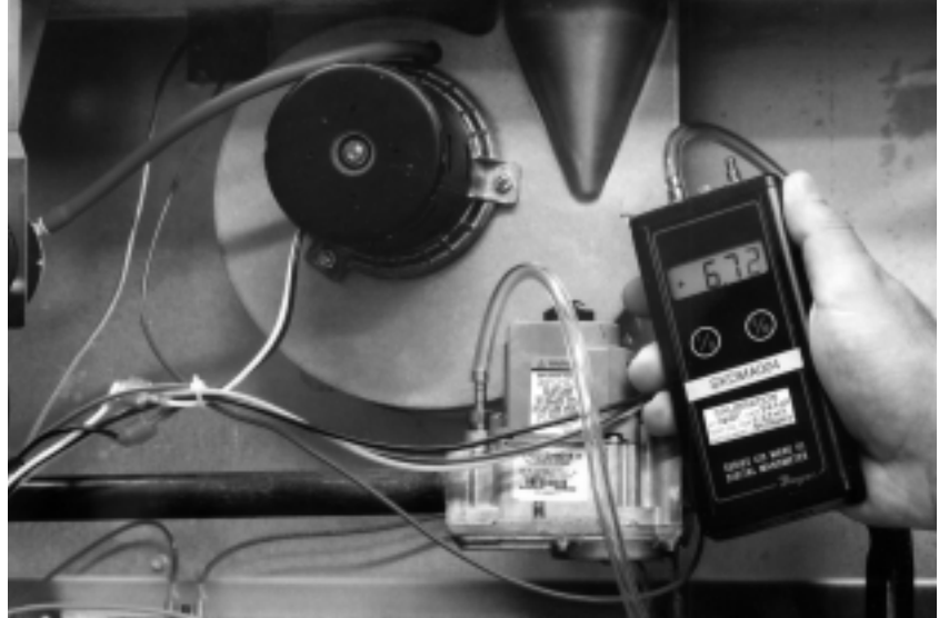
FIGURE 15 TYPICAL HOSE CONNECTION TO LINE PRESSURE TAP
