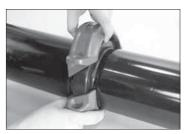
3. **INSTALL HOUSINGS:** Using the "swing-over" feature, install the housings over the gasket. Make sure the housings' keys engage the grooves completely on both pipe ends.
