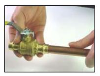
D. Turning slightly, slide press valve on to tubing to the fitting stop. Note: end of tubing must be fully inserted.
