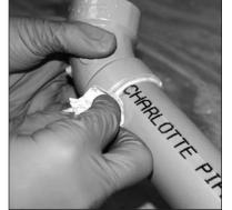
For pipe sizes 6" and larger, two people will be required, a mechanical forcing device should be used and the joint should be held together for up to 3 minutes.
