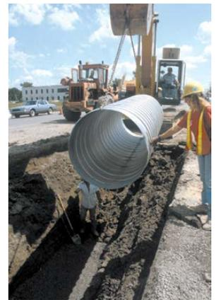
Reduced excavation—because of ULTRA FLO's smaller outside diameter—lowers cost.
