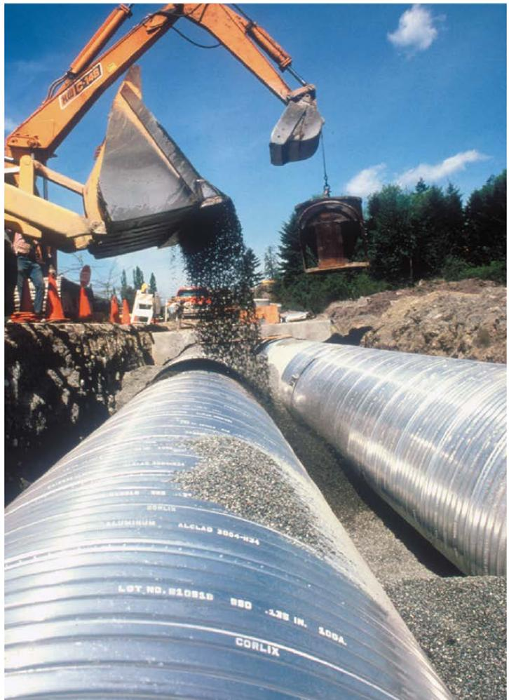
With proper backfilling and cover, CORLIX is an excellent choice for drainage pipe.
