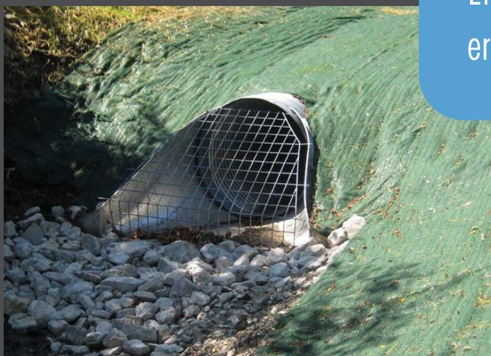
End sections provide protection against erosion and scouring.
