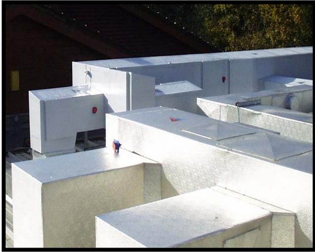
**Venture Tape VentureClad™ 1577CW® is a zero permeability, absolute vapor barrier for insulation cladding and jacketing applications. A 5-ply, self adhesive material installs quickly and easily with no special tools required, resulting in significant time, labor, and cost savings.**
