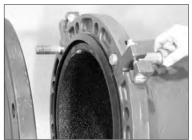
8. INSTALL STANDARD FULL-SHANK-DIAMETER ASSEMBLY BOLTS AT LAP JOINTS: Install a standard full-shank-diameter assembly bolt into each of the lap-joint bolt holes. Refer to the "Helpful Information" table on page 222 for the required assembly bolt size and length. NOTE: Victaulic does not supply these assembly bolts.
