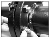
8. INSTALL REMAINING STANDARD FULL-SHANK-DIAMETER ASSEMBLY BOLT/NUTS:
