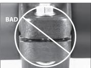
8. Visually inspect each bolt pad location at every joint to verify that full bolt-pad to bolt-pad contact is achieved across the entire bolt pad section.
