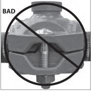
6. Visually inspect the bolt pad location at every joint to verify that metal-to-metal contact is achieved across the entire bolt pad section.
