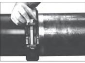
**5. INSTALL BOLTS/NUTS:** Install the bolts, and thread a nut finger-tight onto each bolt. **NOTE:** Verify that the oval neck of each bolt seats properly in the bolt hole.
