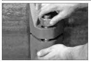
**6a. INSTALL HOUSINGS:** Install the housings over the gasket. Verify that the housings' keys completely engage the groove in each prepared pipe end. Maintain support of the housings while preparing to install the lubricated bolts and nuts.
