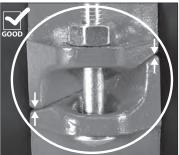
PROPERLY ASSEMBLED JOINT **BOLT PADS WITH EQUAL, NEUTRAL** OFFSETS AT THE BOLT PADS
