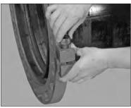
3. INSTALL SECOND SEGMENT: Install the second segment onto the pipe. Install the provided draw bolts into the Style W741, as shown to the left. Thread a provided nut loosely onto each draw bolt. NOTE: The nut should be installed at least flush with the end of the draw bolt but loose enough to permit rotation of the Style W741 for bolt hole alignment in later steps. Verify that the key section of both segments completely engages the groove.
