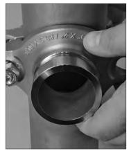
**4. INSTALL HOUSINGS:** Rotate the lower housing so that it is positioned approximately 90° to the upper (outlet) housing, as shown above. The upper (outlet) housing's locating collar shall be placed into the outlet hole. Rotate the lower housing around the pipe.
