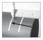
3b. PLACE INSERTION DEPTH MARK ON PIPE/
