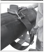
**7. PLACE STRAP:** Push one end of the strap underneath the pipe and hook one U-bolt over the retaining gusset of the spigot housing.
