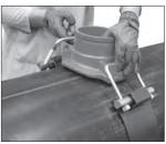
**8. ATTACH STRAP:** On the opposite side of the pipe, pull the second U-bolt up and hook it over the second retaining gusset of the spigot housing. **NOTE:** If there is inadequate length to perform this step, loosen the nuts on the U-bolts to lengthen the assembly.
