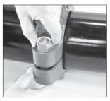
**3. INSTALL BOLTS/NUTS:** Install the bolts, and thread a nut finger-tight onto each bolt.
