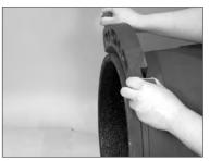
2. INSTALL FIRST SEGMENT: Install the first segment onto the pipe. Verify that the segment's key section completely engages the groove. NOTE: On vertical pipe, the segments shall be supported in place until all segments are installed and fastened together. For horizontal pipe, the first segment can be balanced on top of the pipe, as shown to the left.
