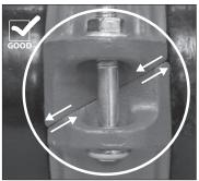
PROPERLY ASSEMBLED JOINT METAL-TO-METAL CONTACT AT ANGLED METAL-TO-METAL CONTACT AT ANGLED BOLT PADS WITH EQUAL, POSITIVE OFFSETS AT THE BOLT PADS
