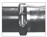
**6. TIGHTEN NUTS:** Using an impact tool or a standard socket wrench with a deep-well socket, tighten the nuts evenly by alternating sides, maintaining nearly uniform bolt pad gaps, until metal-to-metal contact occurs at the bolt pads. Verify that the oval neck of each bolt seats properly in the bolt holes. DO NOT continue to tighten the nuts after the visual, metal-to-metal bolt pad inspection requirement is achieved.
