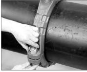
**3a. INSTALL FIRST PRE-ASSEMBLED HALF:** Install the first pre-assembled half over the gasket. Verify that the housings' keys engage the grooves completely on both mating components.
