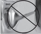
8. Visually inspect each bolt pad location at every joint to verify that metal-to-metal contact is achieved across the entire bolt pad section.
