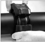
**8. INSTALL HOUSINGS:** Install the housings over the gasket. Verify that the housings' keys engage the grooves completely on both mating components.
