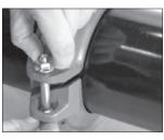
**4. INSTALL REMAINING BOLT/NUT:** Install the remaining bolt, and thread the nut finger-tight onto the bolt. **NOTE:** Verify that the oval neck of each bolt seats properly in the bolt hole.
