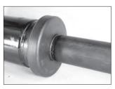
3. JOIN MATING COMPONENTS: Align the centerlines of the two grooved mating component ends and bring them to within the appropriate pipe-end separation dimension. Insert the smaller mating component end into the gasket. NOTE: Verify that no portion of the gasket extends into the groove of either mating component.
