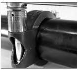
**8. TIGHTEN NUTS:** Using an impact tool or a standard socket wrench with a deep-well socket, tighten the nuts evenly by alternating sides, maintaining nearly uniform bolt pad gaps, until metal-to-metal contact occurs at the bolt pads.
