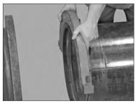
2. INSTALL FIRST SEGMENT: Install the first segment onto the pipe. Verify that the segment's key section completely engages the groove. NOTE: On vertical pipe, the first segment shall be supported in place until the second segment is installed and fastened to the first segment. For horizontal pipe, the first segment can be balanced on top of the pipe, as shown to the left.
