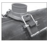
10. TIGHTEN HARDWARE: Using a standard socket wrench with a 1½-inch deep-well socket, tighten both nuts on each U-bolt evenly by alternating between them. Drive one nut no more than ¼ inch/6 mm beyond the location of the second nut on a given U-bolt. To complete the assembly, apply torque to each nut with a torque wrench. Torque the nuts to 75 − 100 ft-lbs/ 102 − 136 N•m, with even spacing between the housing and the strap on both sides. DO NOT exceed 100 ft-lbs/136 N•m of torque on the nuts.
