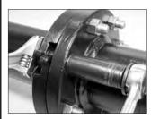
**9. TIGHTEN NUTS:** Tighten all nuts evenly in the applicable pattern shown above until metal-to-metal contact is achieved between the flange faces or the flange-bolt torque requirement for the mating flange is achieved.
