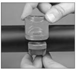
**3a. INSTALL HOUSINGS:** Install the upper (outlet) housing onto the pipe by centering the locating collar in the outlet hole. To check for proper engagement, slide the upper (outlet) housing back and forth while pushing down. A properly positioned upper (outlet) housing will not be able to rotate around the pipe.
