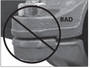
Visually inspect the bolt pad location at every joint to verify that metal-to-metal contact is achieved around the bolt pad perimeter (approximately between the two sets of indicator arrows that are cast into the housings).
