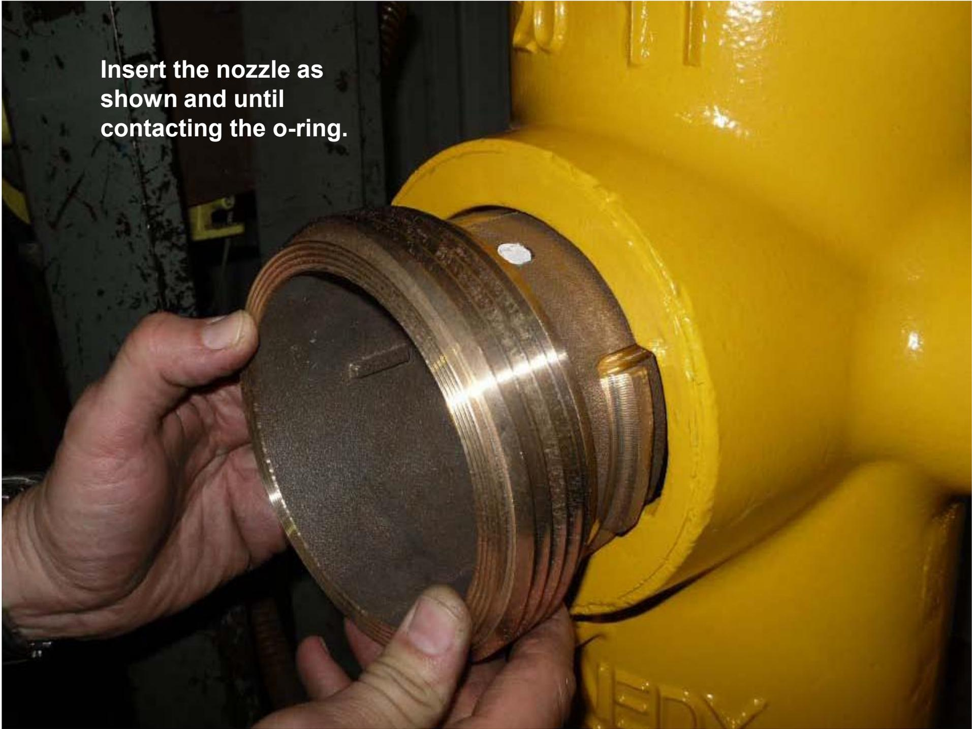
**By hand, rotate the nozzle counter-clockwise as far as possible assuring that the nozzle and the o-ring remain centered.**
