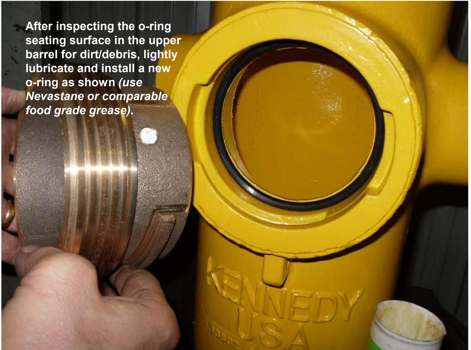
**Insert the nozzle as shown and until contacting the o-ring.**
