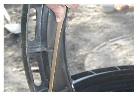
**8.** As before, place the second ring down onto the first with the male lip interlocking into the center of the first ring. For each ring, make sure to line up your paint strip.
