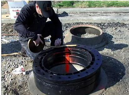
**10.** At this point, you will have all the rings stacked with the sealant applied.
