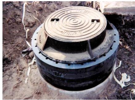
**13.** At this point, the installation of your LADTECH adjustment rings is complete.
