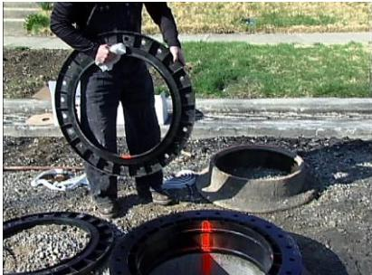
**9.** Repeat the assembly as you did in the prior steps for each additional ring, applying the bead of sealant and placing the rings on top of one another being sure to line up the paint strip.
