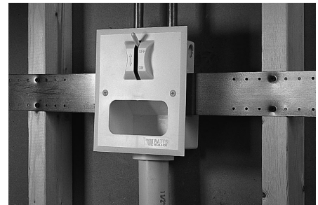
Duo-Clozure wall box roughed in with decorative faceplate installed.
