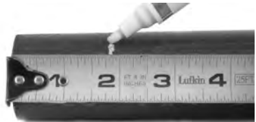
Figure 6A – Marking the Pipe Before Inserting Into Fitting Using Tape Measure
