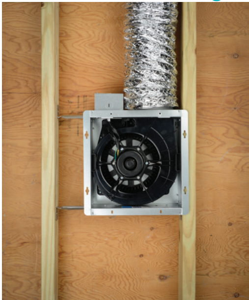
Suitable for sidewall mounting
