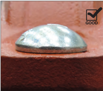
GOOD BOLT ENGAGEMENT (OVAL NECK OF EACH BOLT IS SEATED PROPERLY IN THE BOLT HOLE)
