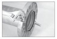
**5a.** Closure lugs are provided to ease installation. Clamp both lugs with a wrench or pliers, and pull the two segments together until the bolt holes align.
