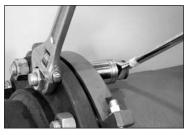
**11. TORQUE FLANGE BOLTS:** Tighten all flange bolts evenly until the required torque value is achieved. Refer to the "Style 341 Torque Requirements" table below for the required torque value.
