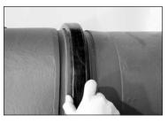
**5. JOIN PIPE ENDS:** Align and bring the two pipe ends together. If the gasket was turned inside out in step 4, roll the gasket into position, and make sure it is centered between the grooves. Make sure no portion of the gasket extends into the groove on either pipe.
