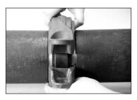
**5. INSTALL HOUSINGS:** Install the housings over the gasket. Make sure the housings' keys engage the grooves properly on both pipes.
