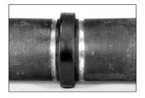
**4. JOIN PIPE ENDS:** Align and bring the two pipe ends together. Slide the gasket into position, and make sure it is centered between the grooves. Make sure no portion of the gasket extends into the groove on either pipe.
