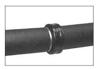
**5. INSTALL GASKET:** Install the gasket onto the plain-end pipe until the pipe end contacts the center leg of the gasket. Insert the grooved pipe end into the gasket until the leading edge of the groove aligns with the outside edge of the gasket.
