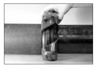
5. INSTALL HOUSINGS: Install the housings over the gasket. Make sure the AWWA markings on the housings face the AWWA pipe. Make sure the housings' keys engage the grooves properly on both pipes.
