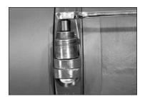
7. TIGHTEN NUTS: Tighten all nuts evenly by alternating sides until metal-to-metal contact occurs at the bolt pads. Make sure the housings' keys completely engage the grooves. NOTE: It is important to tighten all nuts evenly to prevent gasket pinching.
