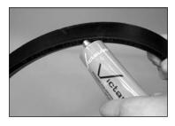
4. CHECK GASKET AND LUBRICATE: Check the gasket to make sure it is suitable for the intended service. Apply a thin coat of Victaulic Lubricant or silicone lubricant to the gasket lips and exterior. NOTE: This gasket is designed to provide the primary seal. Refer to page 43 for special applications.
