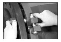
**9.** JOIN VIC-FLANGE ADAPTER AND MATING FLANGE: Guide the four flange bolts, installed in step 7, into the mating flange holes. To prevent the bolts from pulling out, thread a nut finger-tight onto each of the four flange bolts.
