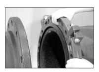
**6.** ALIGN VIC-FLANGE AND MATING FLANGE: Rotate the Vic-Flange on the pipe end, as required, to align the holes with the mating flange.
