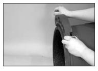
2. ADD FIRST SEGMENT: Place the first segment onto the pipe, making sure the key engages in the groove properly. NOTE: On vertical pipe, the segments must be held in place until all segments are fastened together. For horizontal pipe, the segments can be balanced on top of the pipe, as shown.
