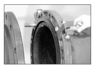
7. INSERT FLANGE BOLTS AT LAP JOINTS: Insert a standard flange bolt into each of the four lap joint holes. NOTE: It may be necessary to tighten the draw bolts to line up the lap joint bolt holes for insertion of the bolts.
