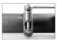
**7. TIGHTEN NUTS:** Tighten all nuts evenly by alternating sides until metal-to-metal contact occurs at the flat bolt pads. **NOTE:** It is important to tighten all nuts evenly to prevent gasket pinching.
