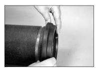
**3. INSTALL GASKET:** Install the larger side of the gasket onto the AWWA pipe end (refer to markings on gasket) until the inner, FlushSeal™ portion of the gasket contacts the pipe end.
