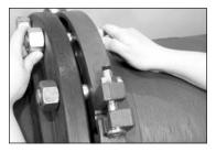
**10.** ADD REMAINING BOLTS/ NUTS: Add the remaining standardflange bolts. Thread nuts finger-tight onto the bolts.
