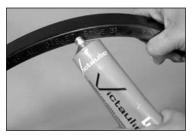
**3.** CHECK GASKET AND LUBRICATE: Check the gasket to make sure it is suitable for the intended service. Apply a thin coat of Victaulic Lubricant or silicone lubricant to the gasket lips and exterior.
