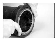
**3. INSTALL GASKET:** Install the gasket over the pipe end. Make sure the gasket does not overhang the pipe end.
