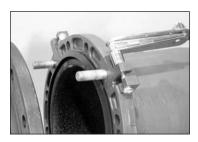
**8.** TIGHTEN DRAW BOLTS: After all four bolts are inserted into the lapjoint bolt holes, torque the draw bolts to approximately 150 ft-lbs (203 N•m). **NOTE:** It is normal to have a small amount of shift as these bolts are being torqued.
