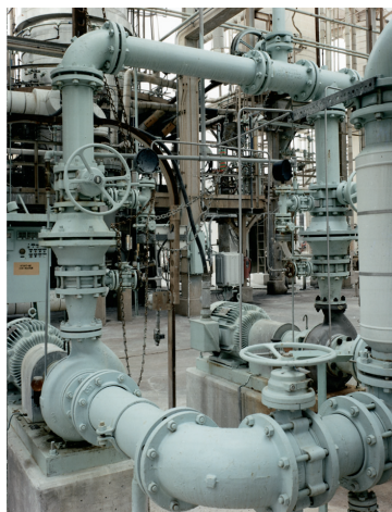
Upper left: C Series spring return actuator with lock-out/tag-out, mounted to a 10" ACRIS isolating a CLO 2 tank in a pulp mill. Upper middle: Manually operated 8" ACRIS replacing plug valves for pump isolation in EDC and VCM service. Upper right: Manually operated 4" ACRIS for UV light isolation in high purity water.
