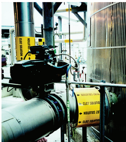
Upper left: C Series spring return actuator with lock-out/tag-out, mounted to a 10" ACRIS isolating a CLO 2 tank in a pulp mill. Upper middle: Manually operated 8" ACRIS replacing plug valves for pump isolation in EDC and VCM service. Upper right: Manually operated 4" ACRIS for UV light isolation in high purity water.
