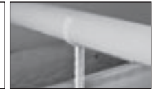
Support horizontal runs of vent pipe in the attic
