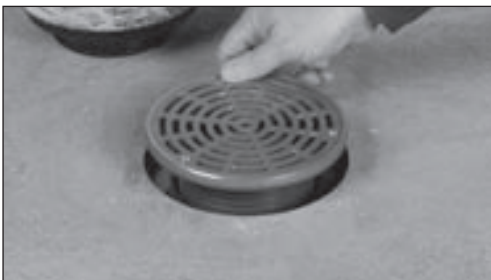
Install Finish Fixture
