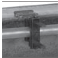
Run pipes parallel to steel I-beams.
