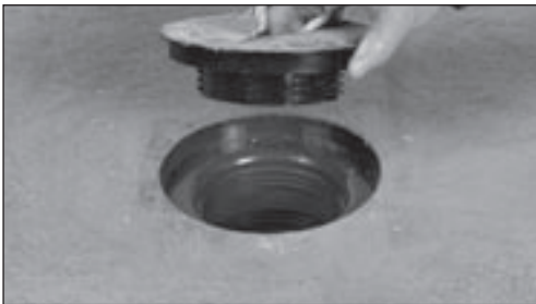
Remove Coring Plug
