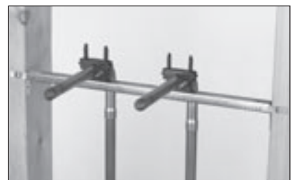
Place tube inside clamps and cinch the bridge down evenly over posts to secure.
