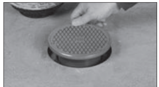
Install Finish Fixture
