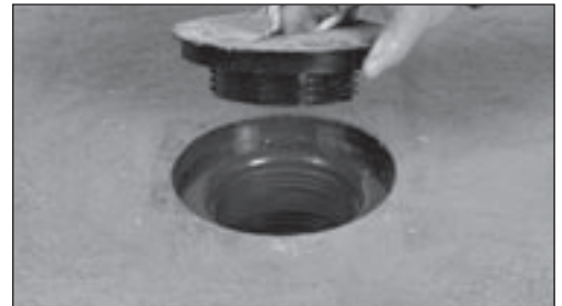
Remove Coring Plug
