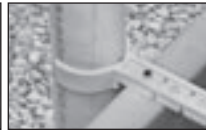
Secure pipe to form for stack placement inside stud wall
