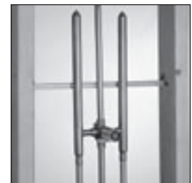
Models with open branches work great for tub valve connections.
