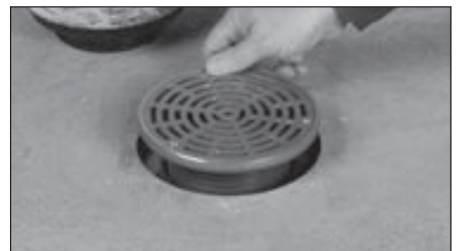
Install Finish Fixture
