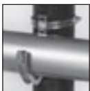
Install on stack or vent pipe
