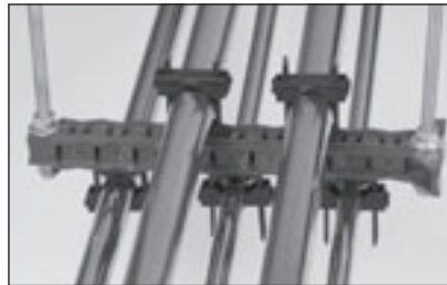
Use 3/8" (#3) threaded rod for trapeze installations.
