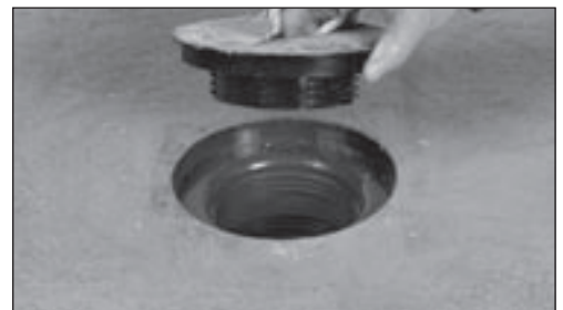
Remove Coring Plug
