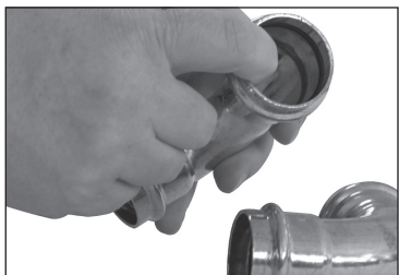
Figure 2 — Check for EPDM Seal
