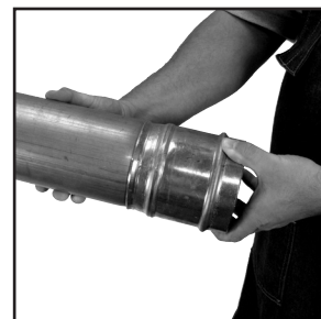
Figure 9: Inspection of final crimp
