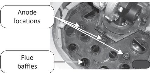
**Note:** EF100T399 models have only 1 anode rod under the 2<sup>nd</sup> pass collector cover.
