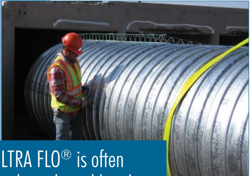
ULTRA FLO® is often used to reline old and deteriorating culverts.
