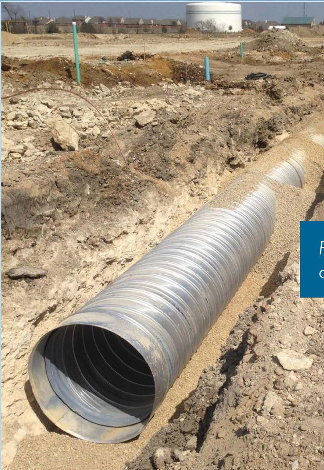
*Proper backfill and placement help ULTRA FLO® achieve its designed structural capacity.*
