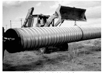
ULTRA FLO® is available in long lengths, and its light weight allows it to be unloaded and handled with small equipment.
