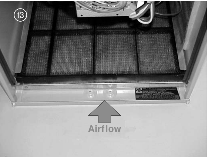
BOTTOM FILTER RACK INSTALLATION
