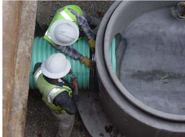
For rubber boot connection two “flat top” gaskets are positioned under the boot to ensure a water tight seal. Manhole boots should be sized to fit the outside diameter of CORR-21.
