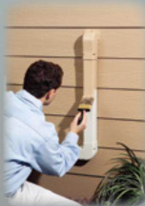
DiversiTech recommends attaching the base to the wall or ceiling and the line sets to the system every 15" to allow for the system to carry the full weight of the line sets.
