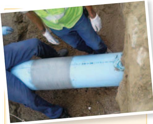
One of the sub-contractors hit the new 12" main water line for the new county building. They left a 10"X12" scratch about 2/3 into the thickness of the pipe, but did not actually pierce it.
