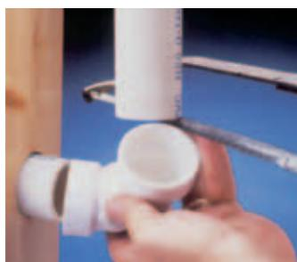
*Damaged or leaking fitting is cut out*
