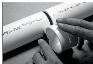
4. Place the repair coupling on the pipe with the larger pipe ID (inside diameter) end facing the gap between the pipe ends.
