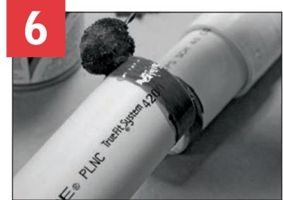
7. Push the repair coupling toward the gap until you reach the mark on the other pipe end. A bead of cement will be present around the entire diameter of the pipe and coupling.
