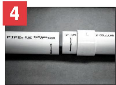
5. Apply primer between the mark and pipe end on both pipe ends. Note: The use of primer for ABS is not recommended. Check local code requirements.
