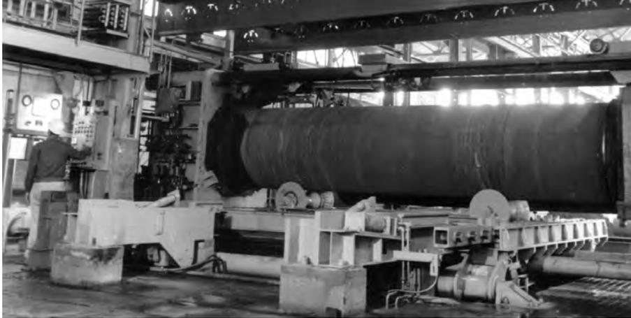
**Each 30" and larger diameter AMERICAN Ductile Iron pipe is hydrostatically tested to 75% of yield strength which results in higher test pressures than those required by AWWA C151, varying to over 900 psi, depending on size and thickness of the pipe.**
