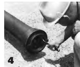
**4.** Firmly install the locking means if needed for restraint in the case of small-diameter Push-On plugs, tighten all cap screws inside the plug, and the assembly is then complete.
