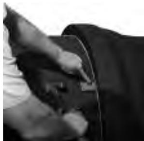
\* Although special disassembly shims can be furnished by AMERICAN upon request, shims of virtually any suitable material, shape, and approximate thickness of the weld height may be used effectively to disassemble the joint.
