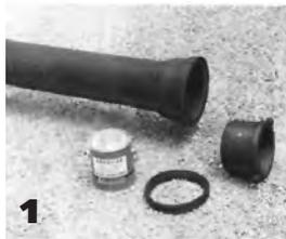
**1.** Clean the pipe socket of any foreign matter and insert the gasket. Lubricate the end of the plug and inside surface of gasket with a thin film of lubricant. A non-soluble lubricant, such as Fastite underwater lubricant, may be used to facilitate removal of the plug after testing.
