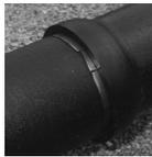
Very tight joints may have to be separated by cutting pipe. The reuse of Fast-Grip gaskets after disassembly is not advised.
