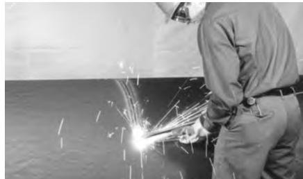
Cutting ductile iron pipe with torch.
