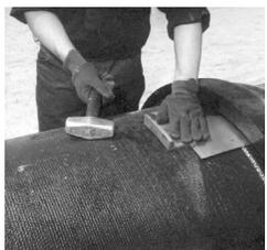
C) Carefully drive a disassembly shim between the gripping teeth of the segments and the spigot with a hammer. Lifting or offsetting of the spigot relative to the socket (to relieve
