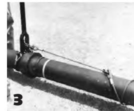
**3.** Larger sizes are easily assembled by placing another pipe against the plug and pushing or pulling the plug "home" using standard Fastite assembly tools or methods.
