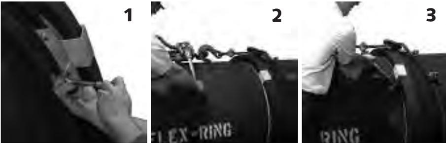
**1.** Remove screws and slotted shipping plate from the segmented ring ends inside the bell. (The Flex-Ring Joint is normally shipped with the joint locking ring in place for assembly.)
