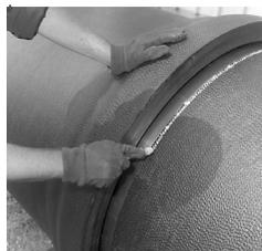
E) After all shims are inserted, place a reference mark on the spigot even with the exposed end of the shims. Pull, jack, or deflect the spigot
