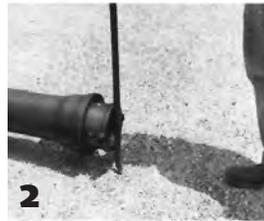
**2.** Place the tapered end of the plug in contact with the gasket in the pipe. Push the plug "home" into the pipe socket with a bar, lever, or jack, as required.
