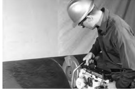
Cutting ductile iron pipe with abrasive wheel.
