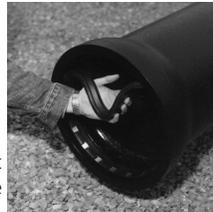
gaskets should be warmed before installing. (One way to keep gaskets warm is to keep them in a truck or heated vehicle cab until they are ready to be used.)
