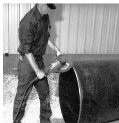
A portable grinder should be used to make a bevel 3/8" to 5/8" long at an angle of 30-40° with the axis of the pipe. All sharp corners or rough edges that might damage or dislodge the Fastite gasket or Field Flex-Ring should be removed from the beveled pipe end.
