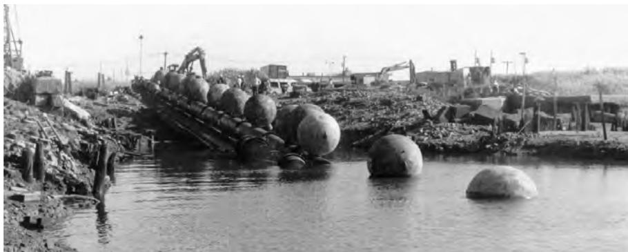
**Flotation provided by attached spheres facilitated installation of this 30" pipeline with Flex-Lok Joints.**
