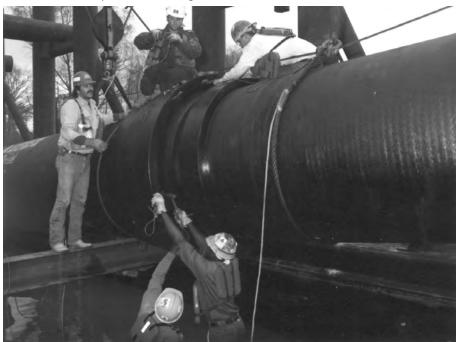
54" AMERICAN Flex-Lok® Joint pipe being assembled for an outfall installation.
