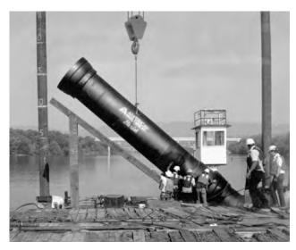
48" Flex-Lok Pipe being positioned for assembly. The ramp attached to the barge is used as the assembly platform, and as the joints are made, the barge is moved forward, allowing assembled piping to slide into the water.
