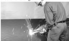
Cutting ductile iron pipe with torch.
