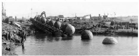
Flotation provided by attached spheres facilitated installation of this 30" pipeline with Flex-
