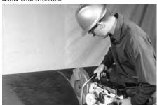
Cutting ductile iron pipe with abrasive wheel.
