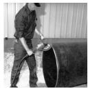
cut as square as possible with the pipe axis and beveled on the outside extreme end after cutting. A portable grinder should be used to make a bevel 3/8" to 5/8" long at an angle of 30-40°
