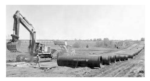
$60^{\prime\prime}$  AMERICAN Fastite  $^{\circ}$  Joint Ductile Iron pipe being installed as a water transmission main.
