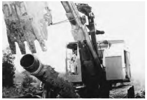
Cast Iron Pipe – being replaced by a larger main – is taken up after years of service for installation in another location for continued service.
