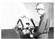
Cutting ductile iron pipe with milling cutter.
