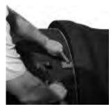
underneath the segments and connecting spring and out of the socket. One shim should be located under the center of the spring to prevent spring deformation or damage during disassembly. Once disassembly shims have been placed (with the pipes in reasonably straight alignment) the spigot should be pulled or jacked out of the socket.
