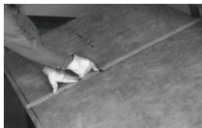
1. Determine board length as described above. Measure and draw groove centerlines starting at left side of board using straightedge, adding stretch-out allowances. Draw two lines for staple flap at right side of board.
