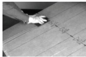
5. Fold up duct and square ends. A folding table makes this job easier. Push out of square and staple flap on about 2" to 3" centers with outward-clinching staples. Start in middle, work toward ends. Release pressure and duct will snap square.
