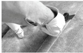
2. Use grey tool to cut female side joint shi lap on left edge of board.
